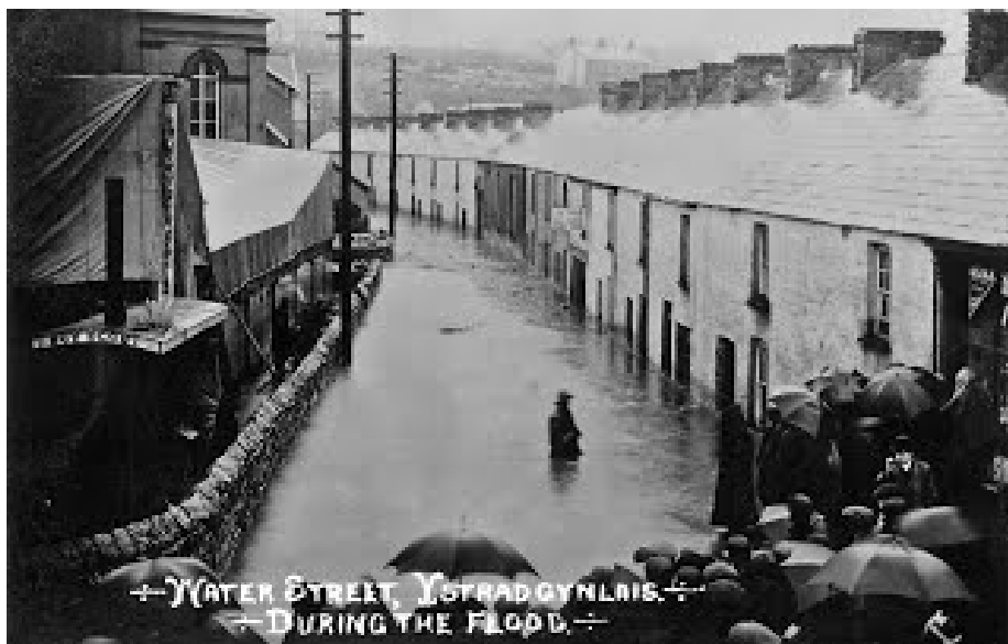
THE SCENE SHOWS WATER STREET YSTRADGYNLAIS DURING THE FLOOD Flood water December 1911
