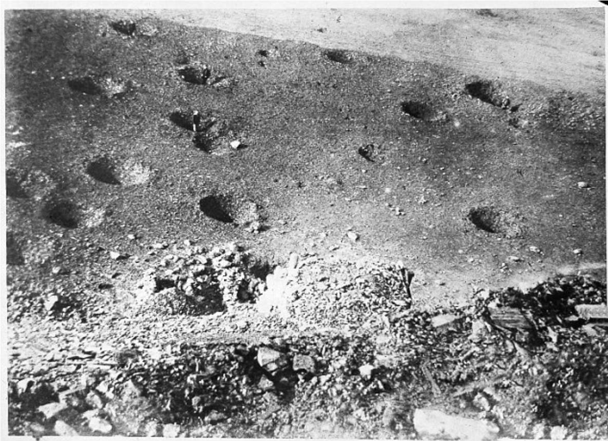
SHELL HOLES ON THE RIDGE
